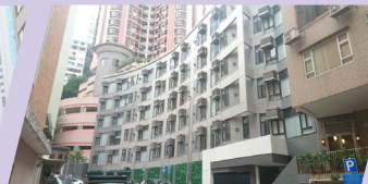
樓宇認證及大型翻新後外觀 Building façade after renovation
