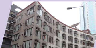
樓宇認證及大型翻新前外觀 Building façade before renovation
