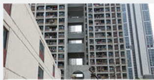
祈德尊新邨 (荃灣) C 座、松明舍、商場、幼稚園大樓及公用設施 Clague Garden Estate (Tsuen Wan) Tower C, Chung Ming Sheh, Commercial Complex, Kindergarten and Nursery Building and Utilities Blocks
